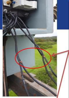
The disconnection of the CT/VT wiring at the terminal box was done by the CNC.
