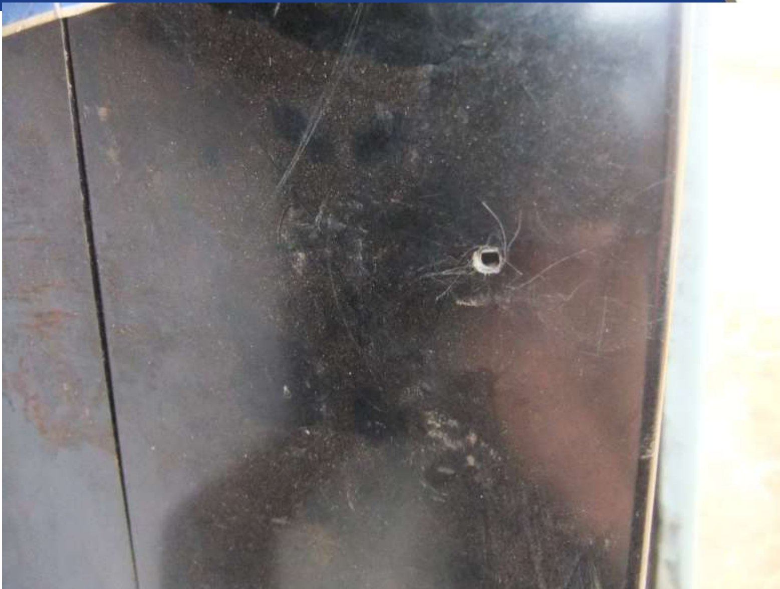
Hole drilled in side of meter
