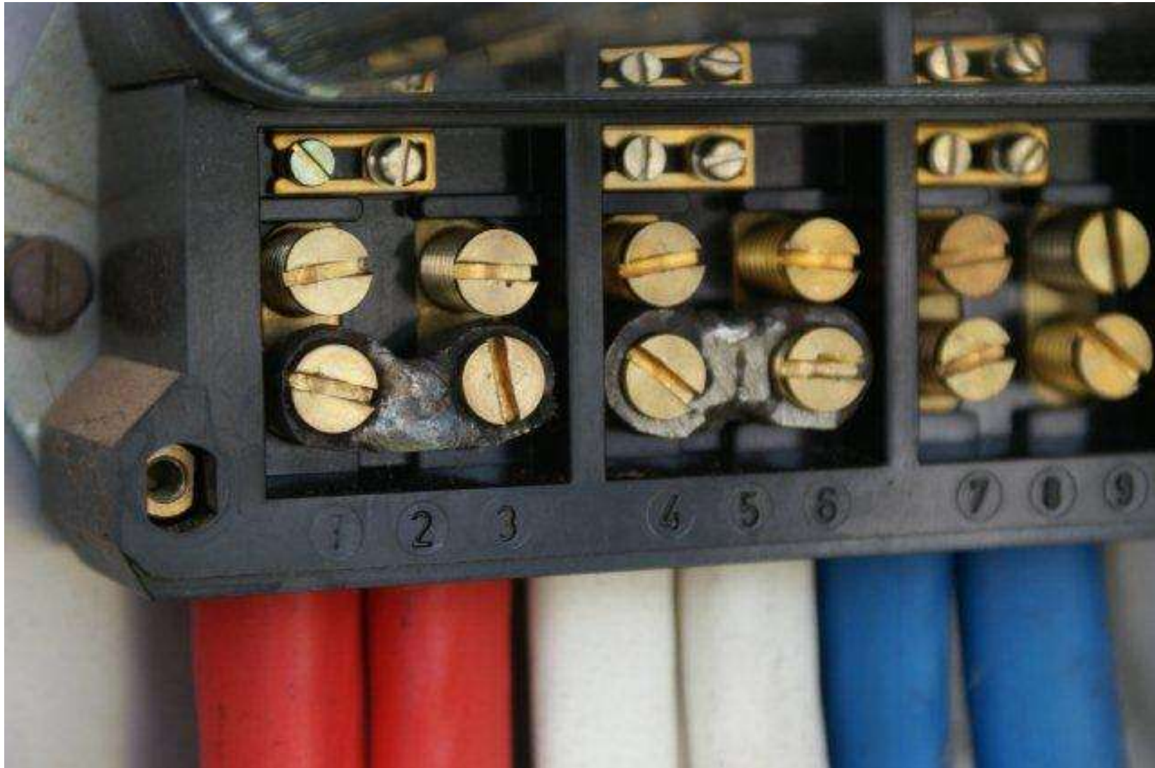
Bridge between line and load
