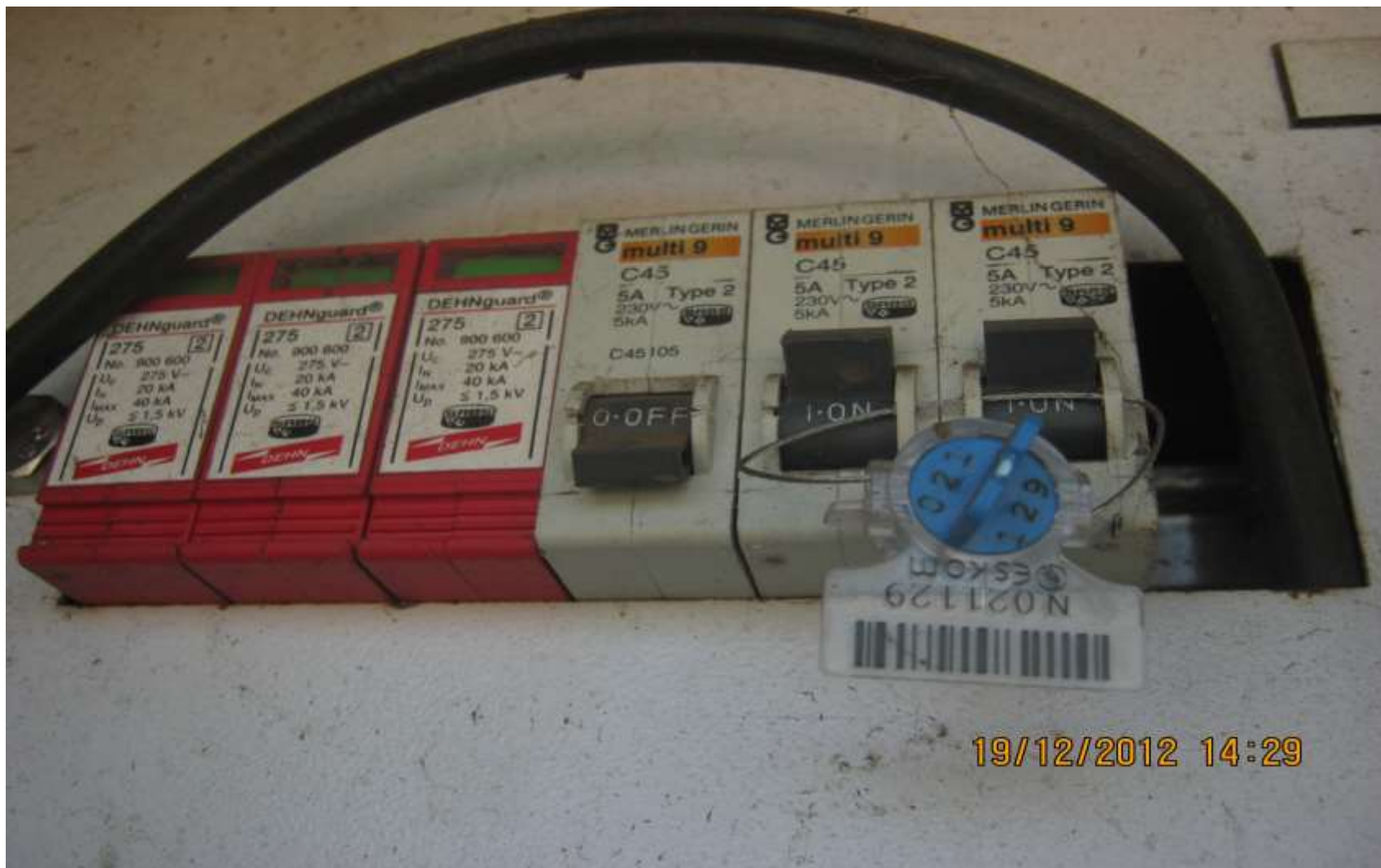
Metering circuit breaker switched off
