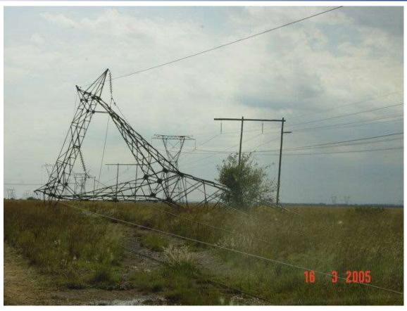
Losses suffered as a result of one line that collapses as a result of theft of steal lattices could amount to more than what Eskom lose as a result of conductor theft in a year.
