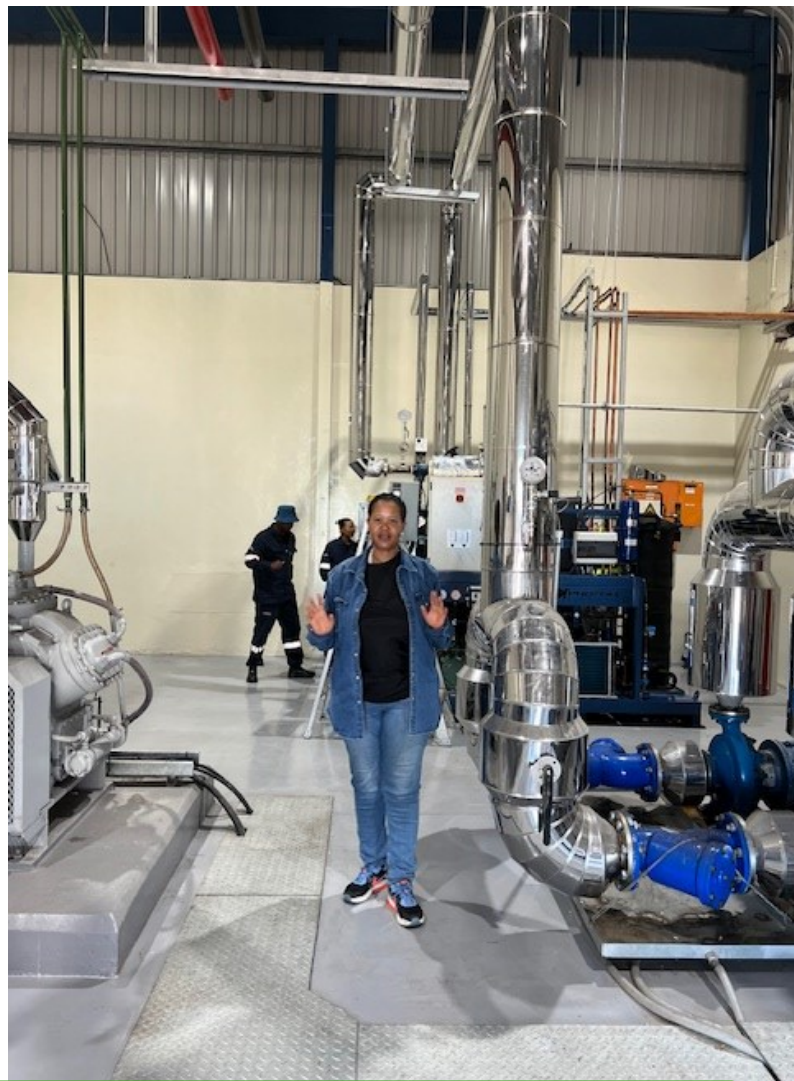
R717/744 Cascade system of full CO2 and ammonia installed
