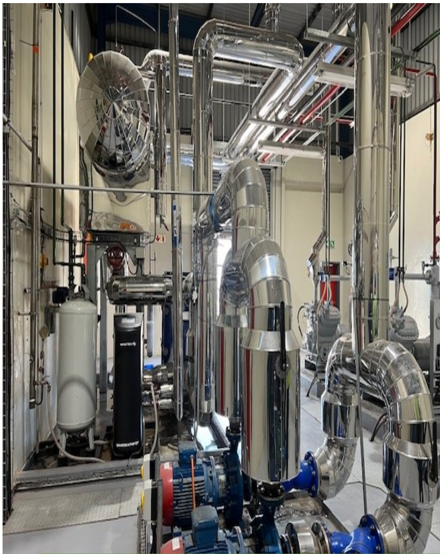
R717/744 Cascade system of full CO2 and ammonia installed
