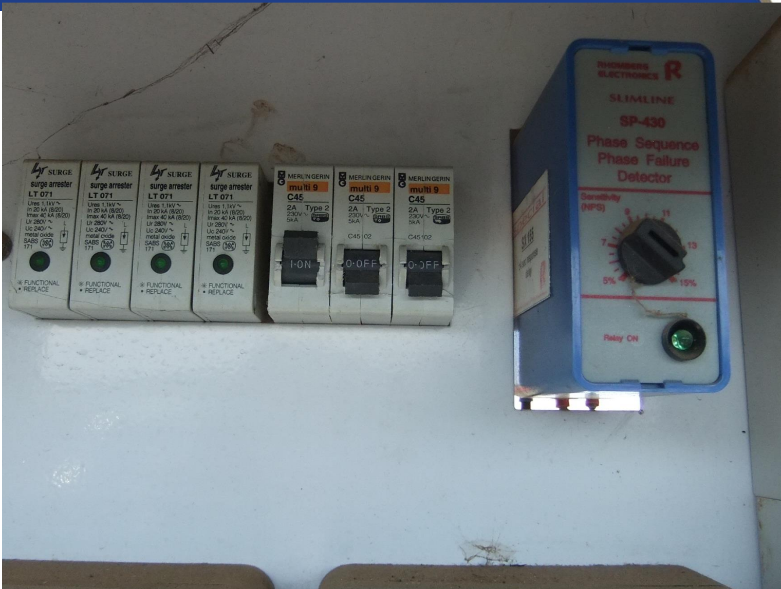
Metering circuit breaker switched off
