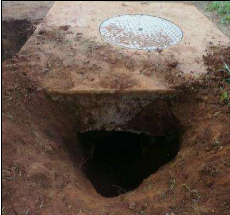
Breaking into a manhole from the side
