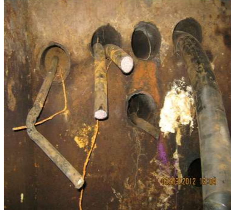
Cables cut in a manhole
